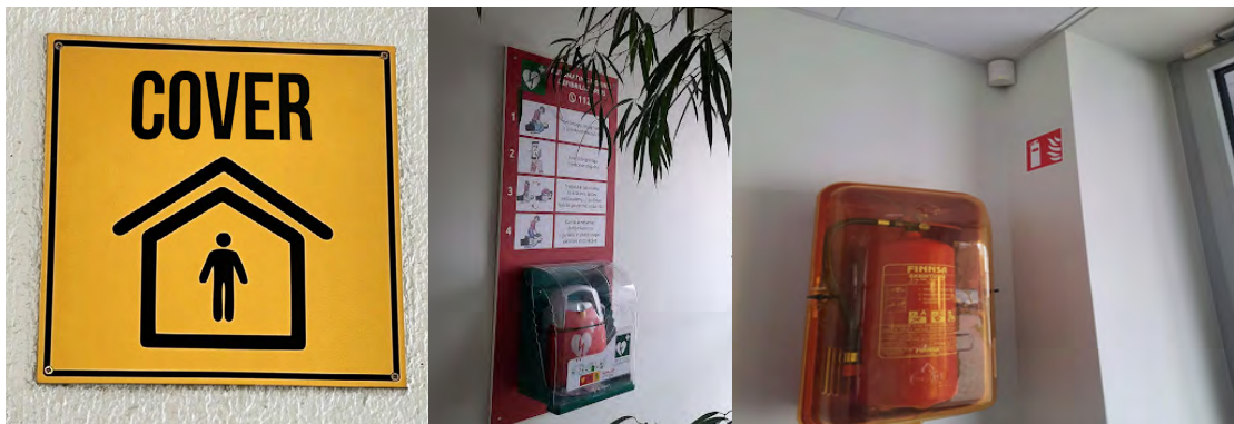
Figure 43 Examples of security infrastructure
