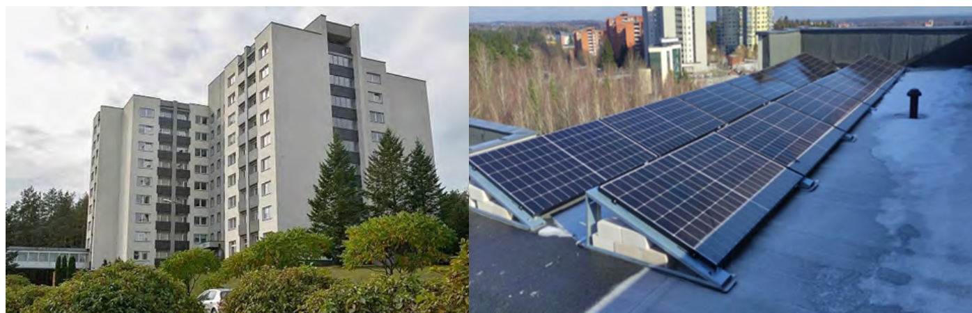
Figure 40 Solar power plant on the roof of the MRU Student Dormitory
